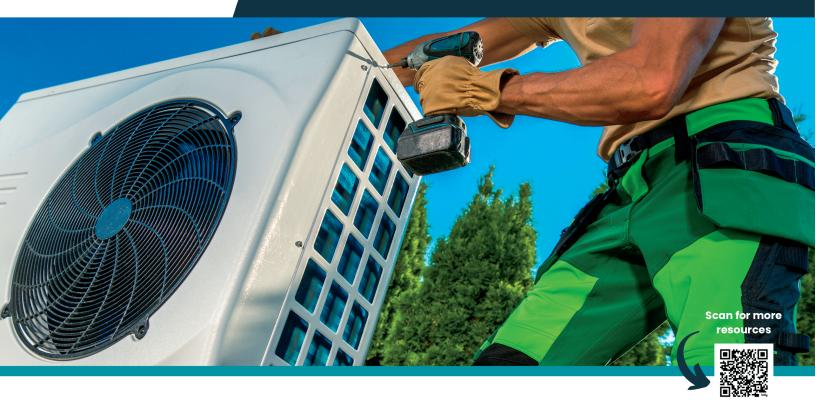
Heat pump water heaters are devices that efficiently heat water by transferring heat from the air or ground rather than generating it directly. They use electricity to move heat, typically drawing in ambient air, extracting heat, and warming water in a storage tank. This technology significantly lowers energy consumption and utility bills while providing a consistent supply of hot water.
