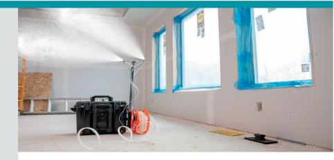
The home is prepared by covering all unsealed openings and surfaces. The blower door system then pressurizes the space, with a computer controlling the temperature, pressure, humidity, and sealant distribution.
