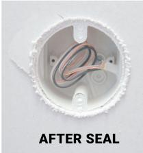
Sealing stations begin spraying atomized sealant. The sealant follows air currents through air leaks and seals them.
